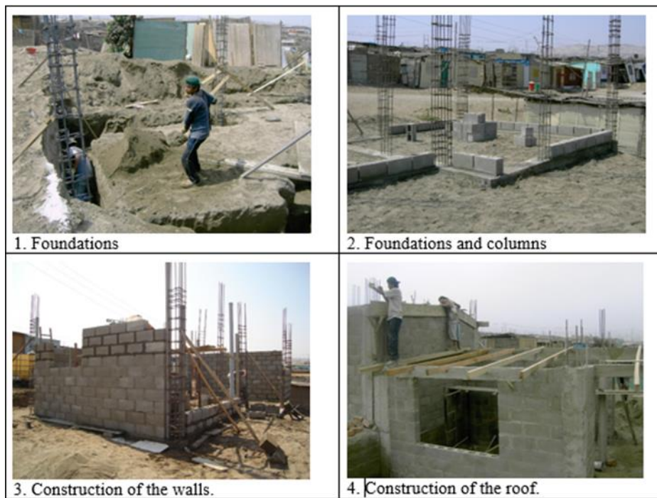
Figure 11 Concrete structures for houses to be earthquake resistant
